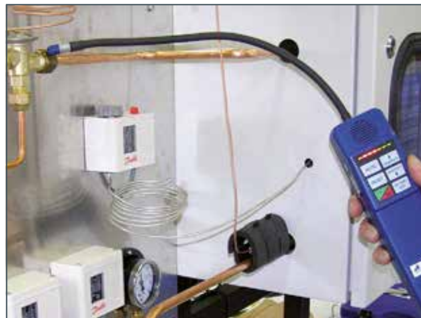
Leak testing at expansion valve
